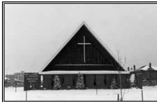
Before the renovation
